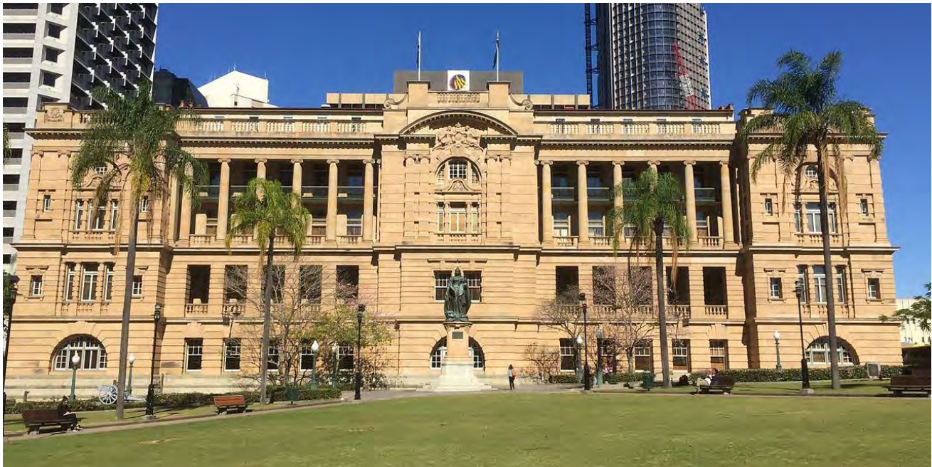
Lands Administration Building [Elizabeth, William, and George Streets]
